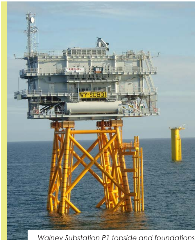
Walney Substation P1 topside and foundations
