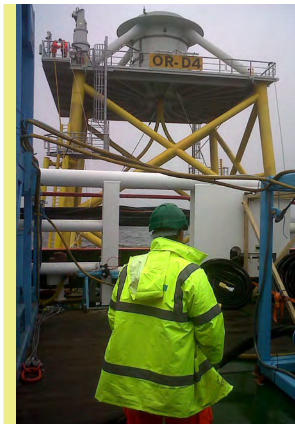
FoundOcean offshore crew looking out over the jacket whilst the grout hose is being moved to the next top-side grout connector
