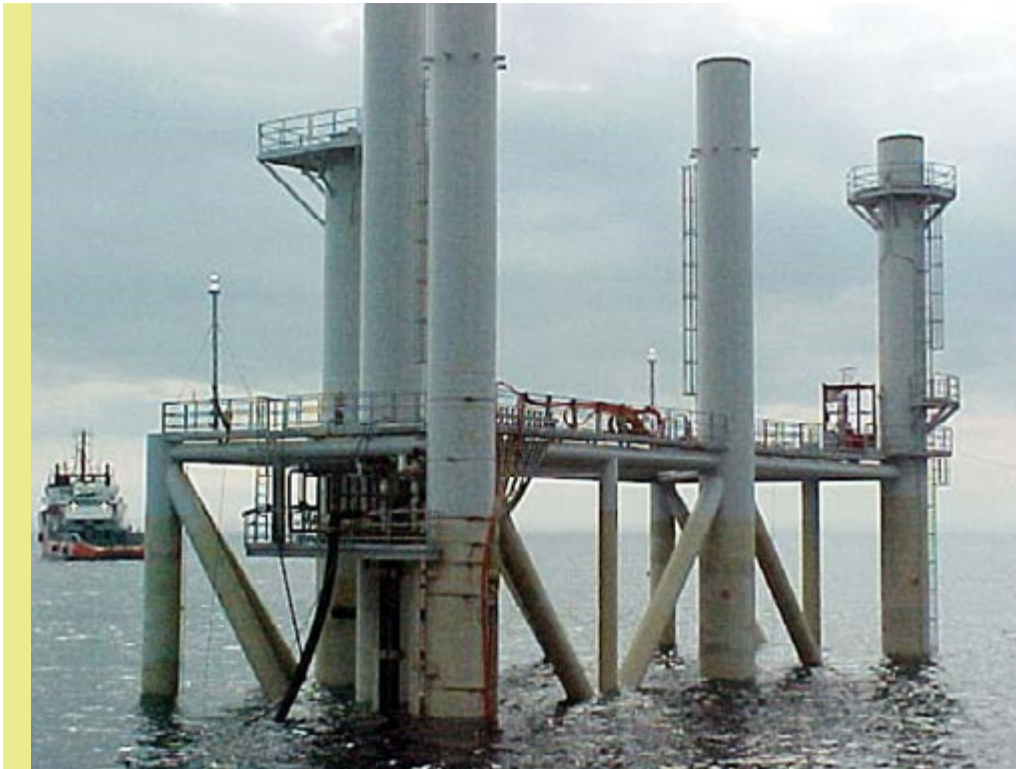
The Hanze F2A Gravity Base Structure in situ
