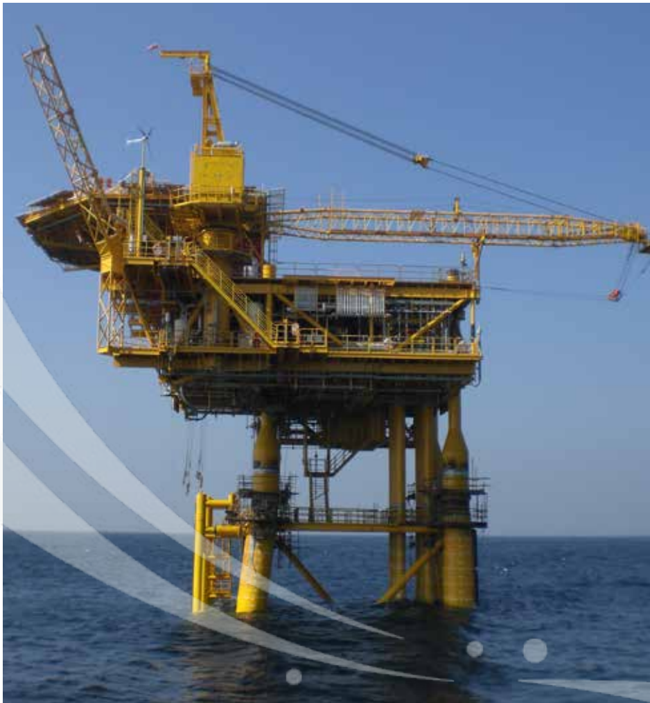
© FoundOcean 2013 - Cluster 7 Wellhead Platform
