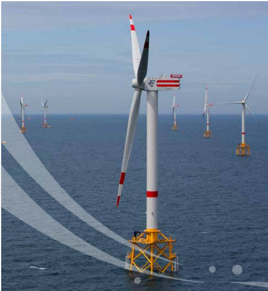
© C-Power 2013 - Thornton Bank Offshore Wind Farm
