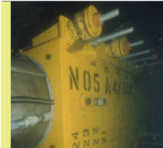
Grouted clamp in situ
