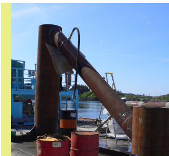
Member grout filling trials
