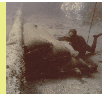
Diver installed formwork
